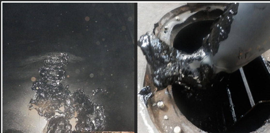
Wax deposition in man hole
