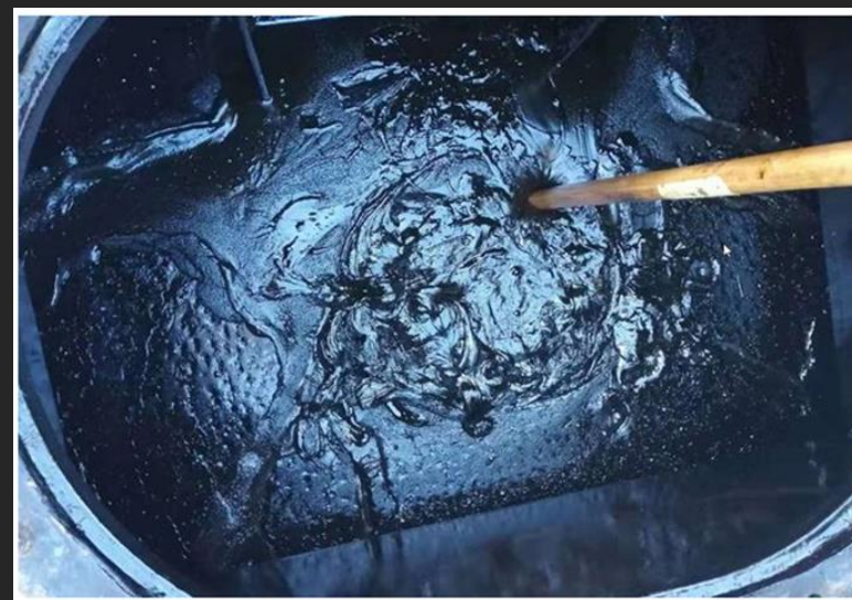
Fuel solidification and wax deposition in a storage tank (btm)
